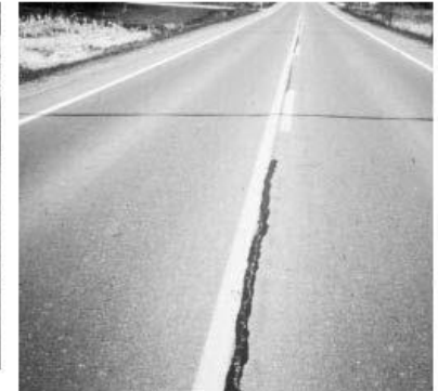
▼ Widely spaced, sealed cracks.
