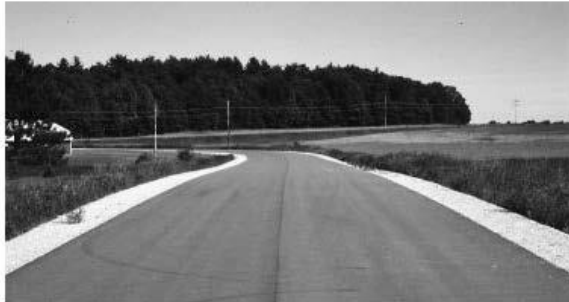
▶ RATING 10 New construction.
