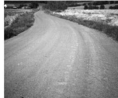
▲ New cold mix surface.
