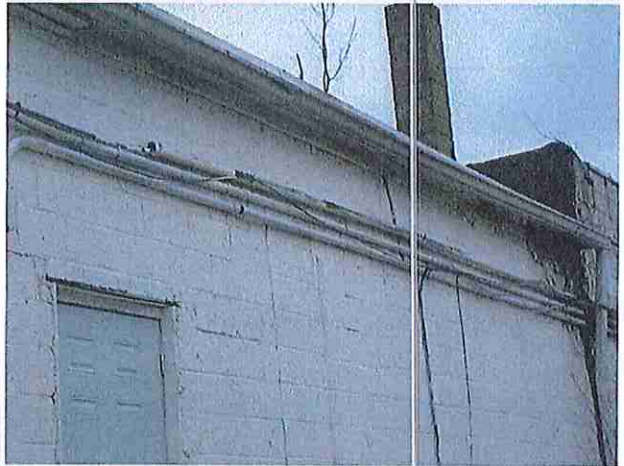
Gutters we are replacing
