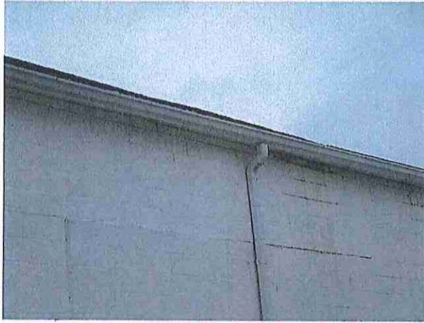
Gutters we are replacing
