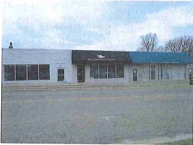
Front of building w/ 3 units
